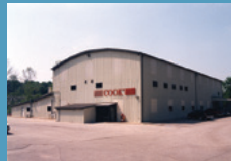
Ellettsville West, Ellettsville, Indiana: a Cook machine shop supporting manufacturing by creating tooling, modifying parts, and preparing materials for manufacturing
